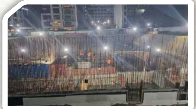
Stair, Lift Core, Shear wall 2nd lift Casting
